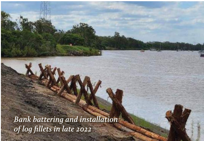
Bank battering and installation of log fillets in late 2022
